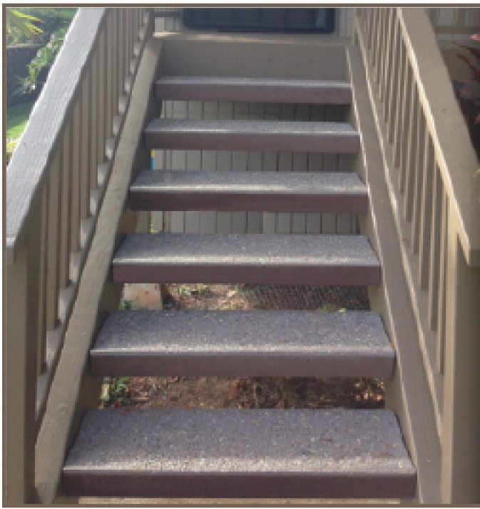
Above & Below: AFTER replacing the 20 year treads & stringers. Above: BEFORE
