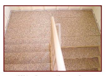
180° Landings provide a seemless appearance. Factory blockouts eliminate any cutting on site for posts. Consulting with us on landings during the design stage will save a lot of time & money!
