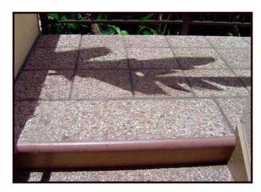
These paver tiles are 1" X 12"X 12", thinset over concrete board. "Expresso" color and exposed aggregate matches the Steptreads. They replaced uninviting worn carpet and rotten landings.
