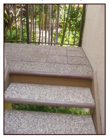
These paver tiles are 1" X 12"X 12", thinset over concrete board. "Expresso" color and exposed aggregate matches the Steptreads. A nosing tread transitions to the landing from below.
