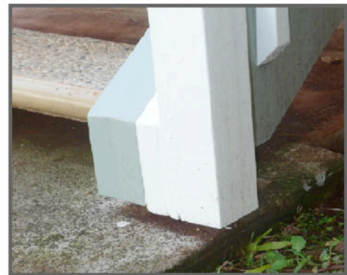
Below is "After", with new posts and stringers suspended on treated brackets. Is this overkill? The fastening method at left has lasted 20 years.
