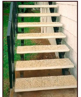
**Wailuna Townhouses** in Pearl City Hts, Oahu. 800 Treads were installed 11 years ago to replace corroded contractor-made concrete treads. Res.Mgr. Norm Hangman installed them in-house.(456-1215)
