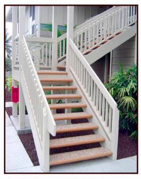
Construction covers eliminate temporaries during construction, then are removed after final painting.
